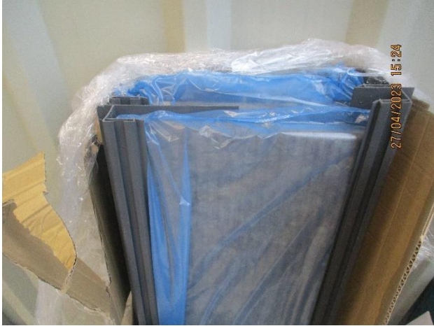
Cavity barrier with plastic extrusion and film
