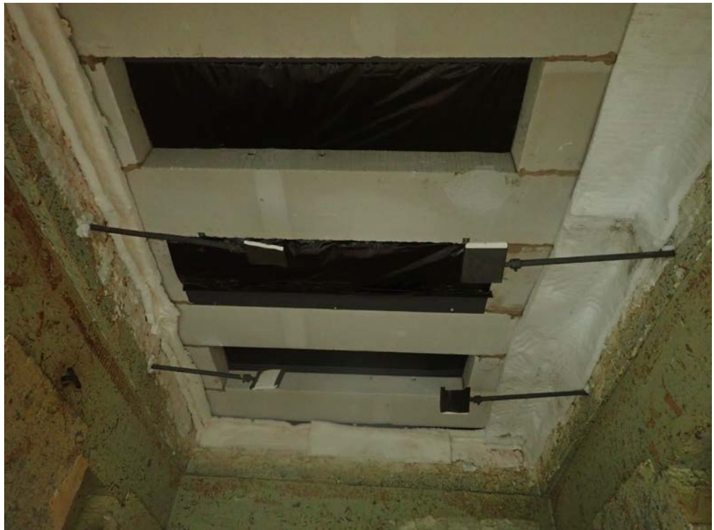
The exposed face of the horizontal assembly prior to testing
